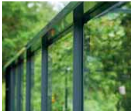
Plastic mouldings – are used for the mounting of toughened glass and polycarbonate glazing, and beautifully unify the overall style.
